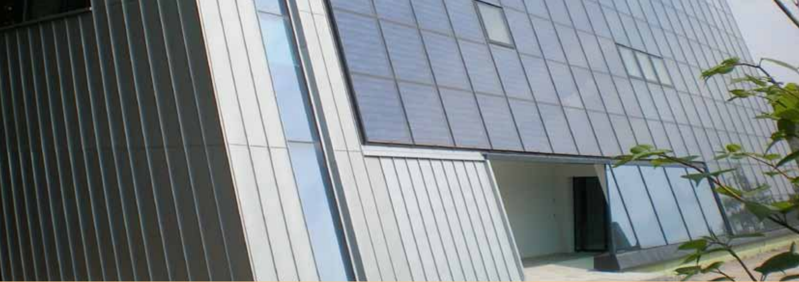
Figure 1: Energy-optimized office building on the basis of a holistic integrated energy management concept / © FASA AG ENERGETIKhaus100 office
